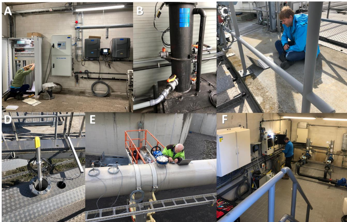
Fig. 1 Impression of the research lane at WWTP Amsterdam West. (A) Research room under primary settler for influent and Nitrous Oxide (N 2 O) measurements; (B) Influent flow-through vessel (C and D) Installation of sensors in the Aeration Tank (AT); (E) Installation process airflow measurement ; (F) Effluent analyzers.
