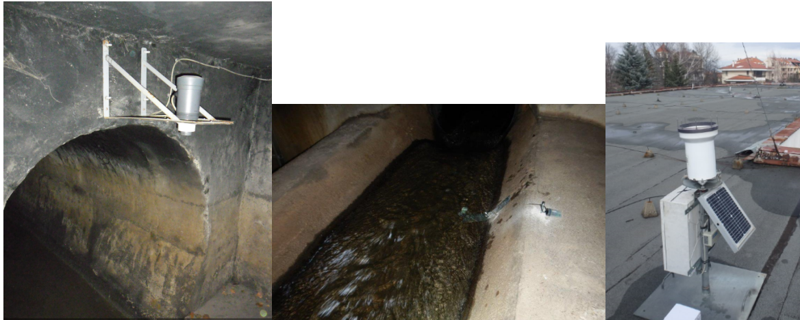
Figure 2: Installation of the water sensor
